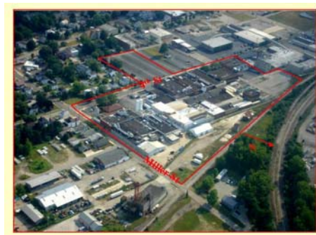
Hospira site on 4th Street before Demolition
